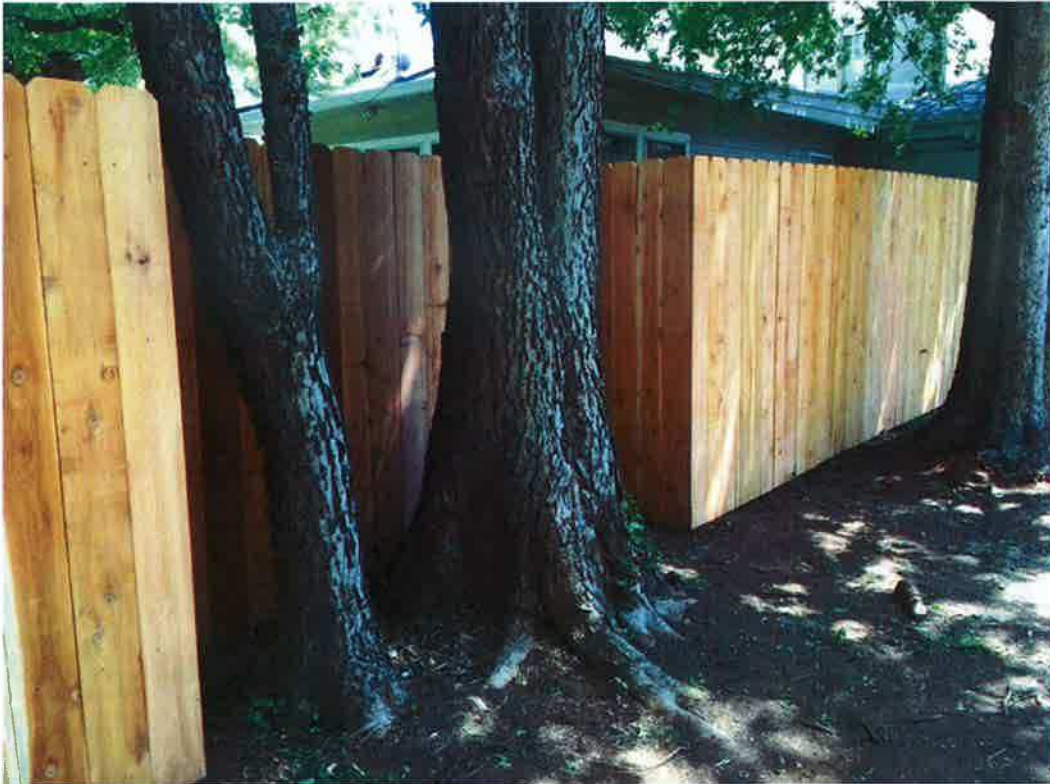
Figure 2: An example of a fence constructed around a tree
